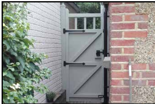
Access gate to back gardens, that provides a clear route for refuse bins to be moved from back gardens to the front of the property for collection
