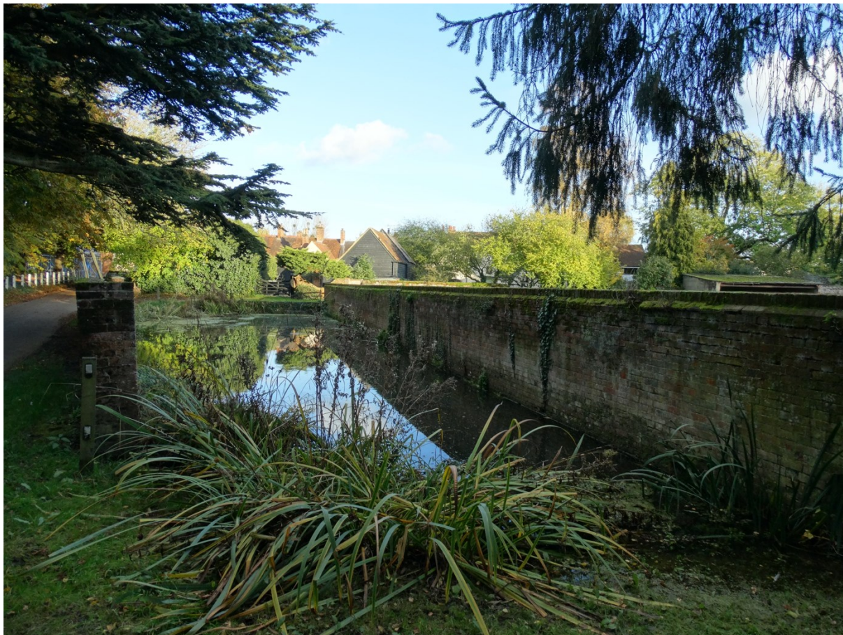
Figure 11: Barkway Carriage Wash (Grade II Listed)
