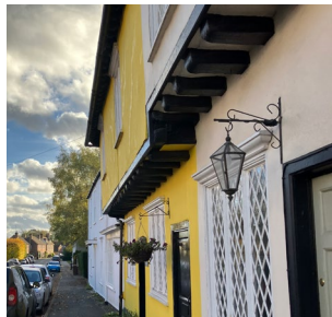
Exposed, black painted timber joists
