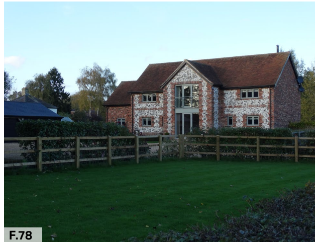
Figure 78: Flint and brick new build property in Barkway.
