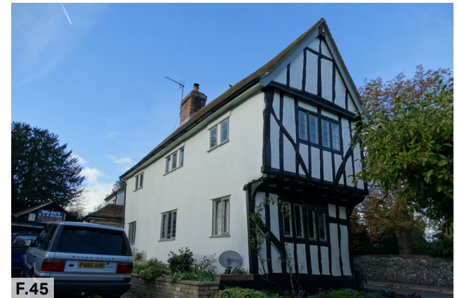
Figure 45: Grade II* listed building at the top of Barkway High Street.
