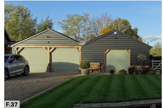
Figure 37: Garages on Highfield Grove, with weatherboarding and timber.
