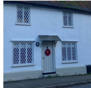
Pentice porch with slate roof
