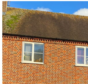
Brick dentil course under the roof eaves
