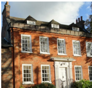
Pitched roof with stone coped gable end parapets
