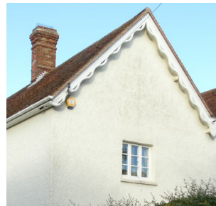
Detailing under roof eaves
