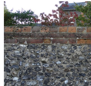
Flint and brick wall
