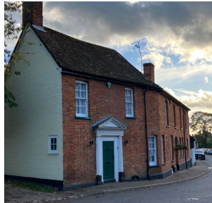
Pitched roof porch with columns and detailing
