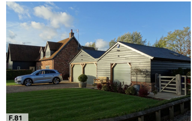
Figure 81: Use of agricultural style outbuildings as garages with pitched roofs, weatherboarding and timber.
