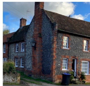
Red brick dressing on flint walls
