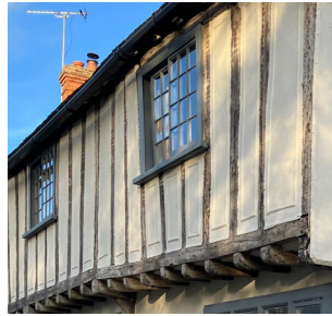
Exposed timber joists under jettied first floor
