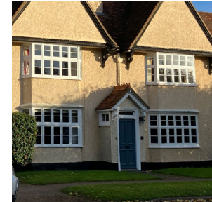
Clay tiled, pitched roof, enclosed porch with detailing
