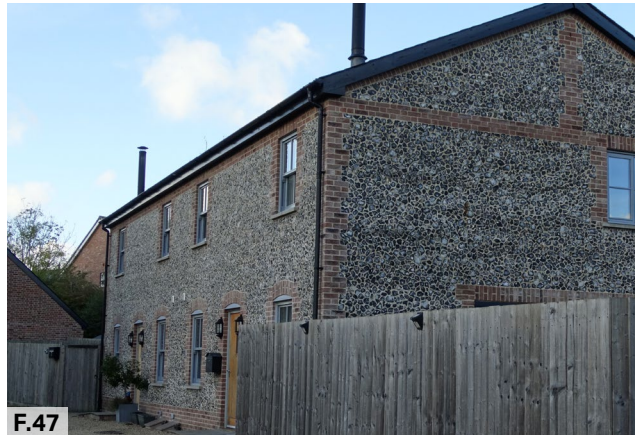
Figure 47: Infill development on the High Street in flint with red brick dressing which references the nearby, older flint building.
