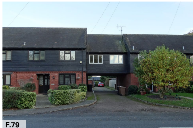
Figure 79: Brick and weatherboarding modern building in Barkway using coach house style influence in its design.
