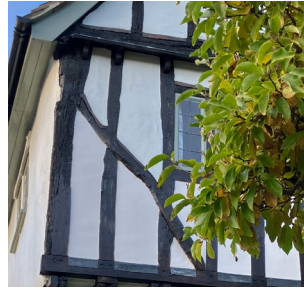
Exposed timber framing
