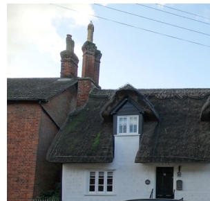
Tall brick chimney stack
