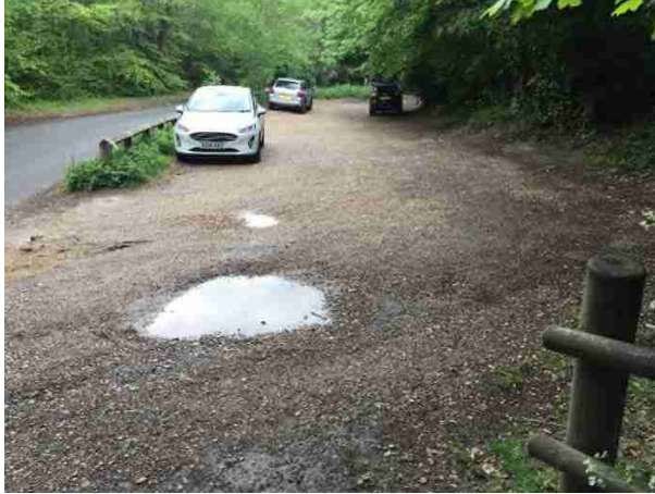
Potholes in Chalk Hills car park
