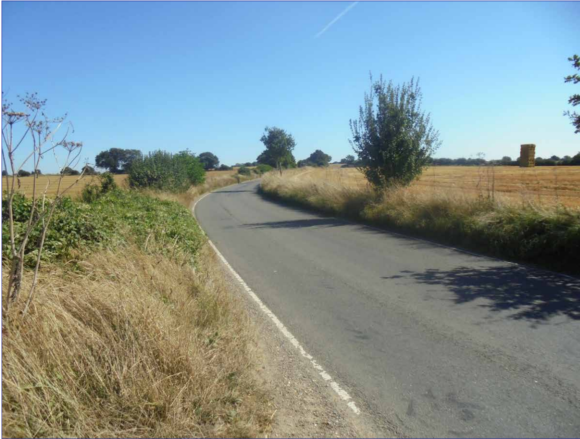
Plate 1: East-facing view along Graveley Lane separating the two parts of the Site
