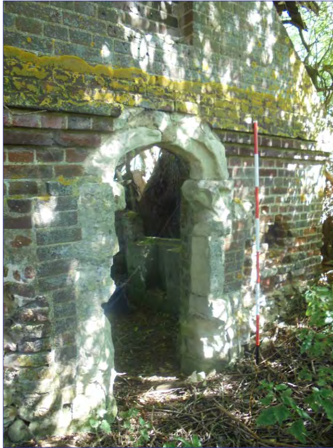
Plate 23: Detail of medieval archway within conduit head building (Site 77)
