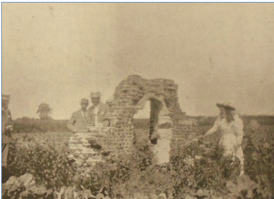
Archive Photograph 4: Undated photograph of the ruined conduit head held in the Gerish Collection, c. late-19 th century (reproduced from Hertfordshire Archives: D/G1/87/2/20)
