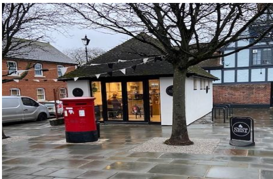
Converted toilet, Lower King Street, Royston
