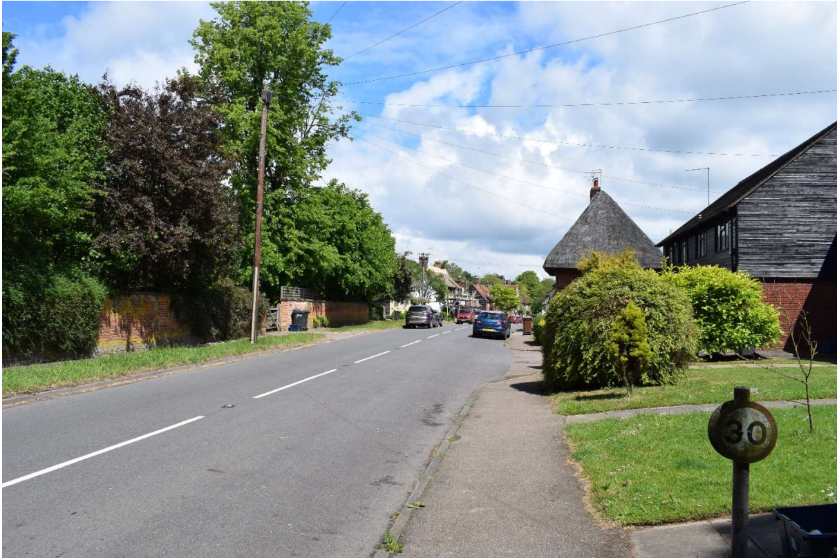
KV8: View from High Street adjacent to the entrance to Ashgrove looking north. This illustrates the linear form of High Street from the south.
