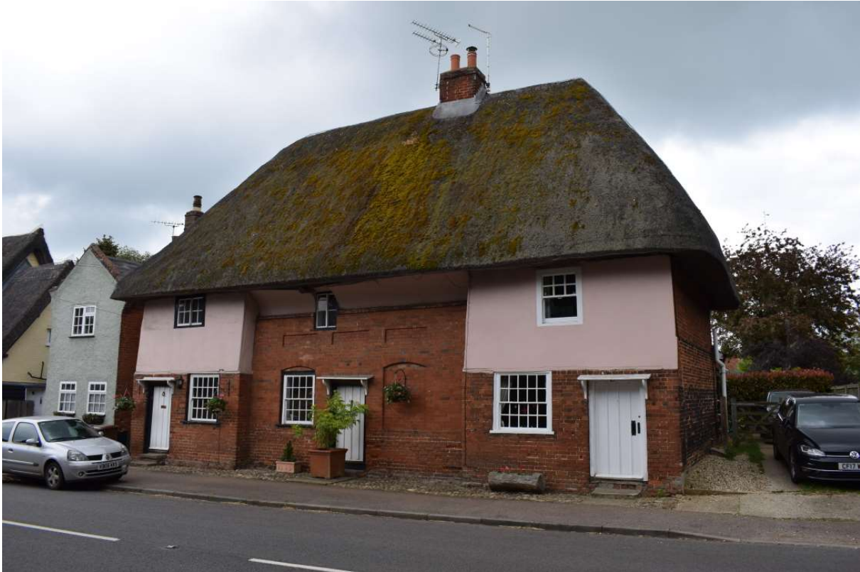
Figure 2.1 The late 15th century 93/95 and 97 High Street (1174330), an example of a Wealden house that has been partly encased in brick (looking east).
